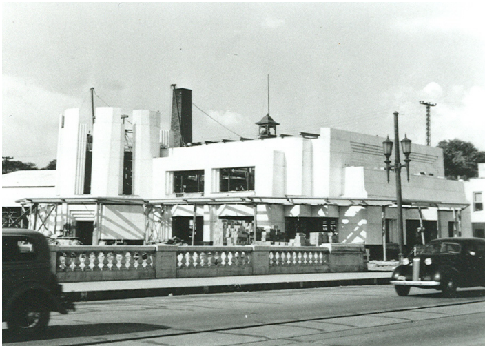
The St. Charles Municipal Building under construction in 1939.
